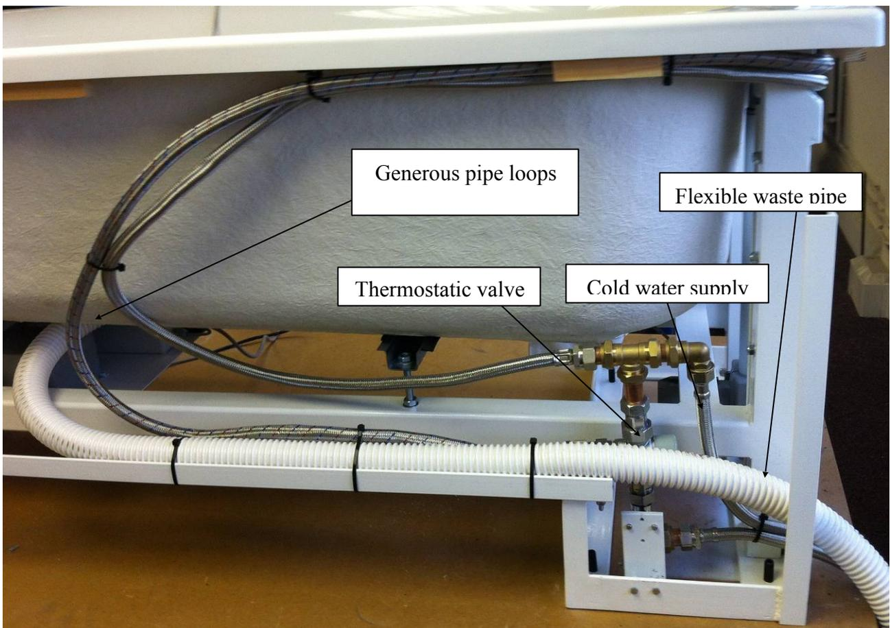
If pipe-work is not supplied, or the installation is modified, it is important to ensure that the above layout is maintained, with generous pipe loops to ensure that the pipe-work is not under any strain during raising and lowering of the bath. These should be positioned in the space along the side of the bath, between the bath wall and the panels.
