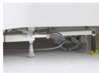
Electronic box sits neatly into metal brackets under bath for access. Magnets plinth brackets
